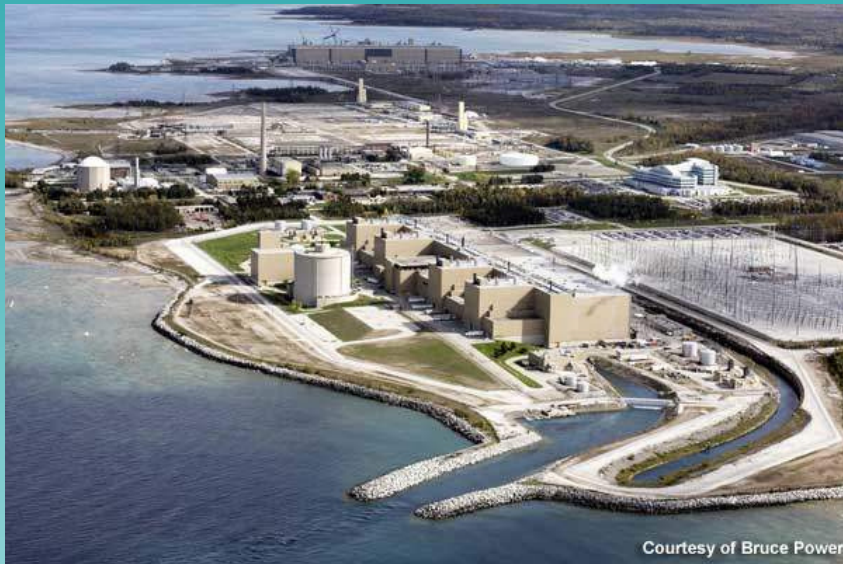
Bruce Power Generating Station, Tiverton, ON, credit: Bruce Power
